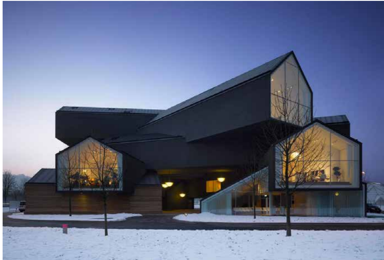
Figure 4-12: Vitrahouse, Herzog and de Meuron, 2006
